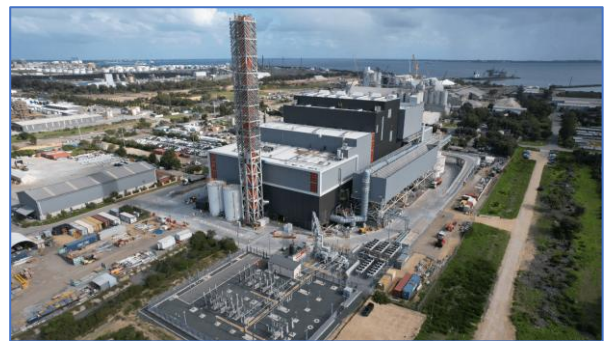
Figure 2 Kwinana Energy Recovery Facility Source: Ramboll
